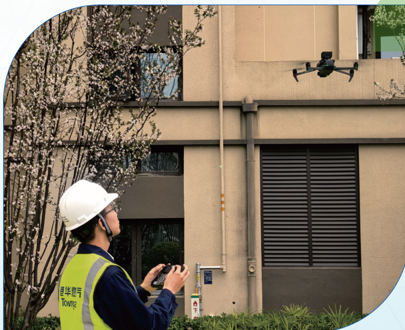
Drones are used to inspect riser pipes in residential areas, as this improves management efficiency and helps ensure community safety.
