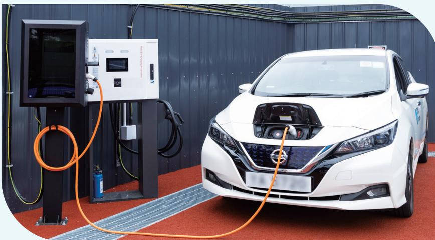
In a trial project in Sai Kung, hydrogen is extracted from the town gas network to power hydrogen fuel cell for EV charging.
