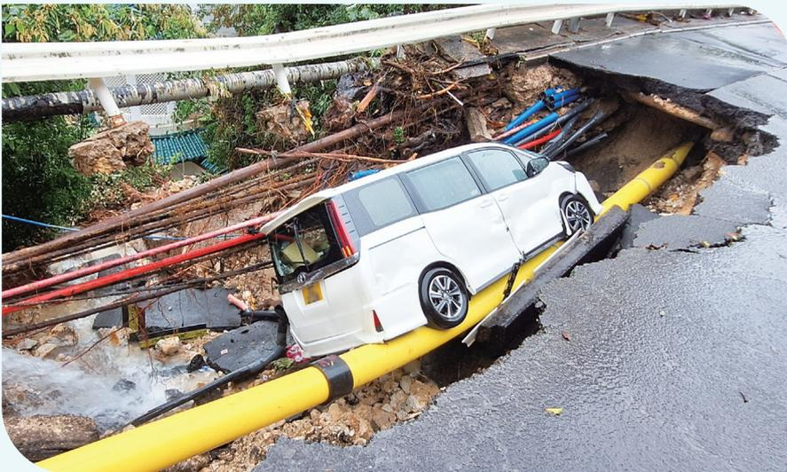
This car fell into a sinkhole near Repulse Bay during the severe rainstorm on 8 September 2023. The gas pipe and joint under the car remained intact thanks to Towngas' meticulous workmanship.
