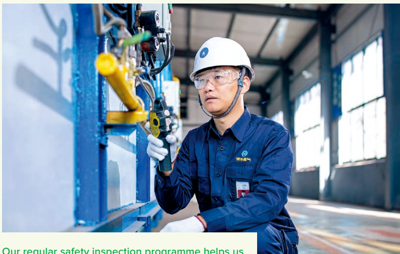
Our regular safety inspection programme helps us maintain the highest standard of customer safety.
