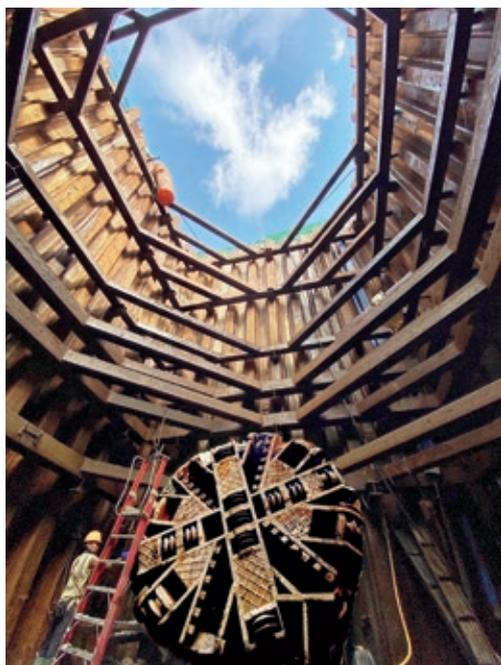
U-Tech's advanced trenchless approach to tunnel boring is being used to install cooling pipes for the District Cooling System at Kai Tak Development Area.
