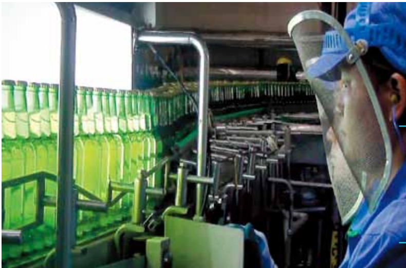
A brewery in Jinan, Shandong province, utilises steam generated by natural gas boilers not only in the process of barley fermentation, but also to clean and sanitise beer bottles.
