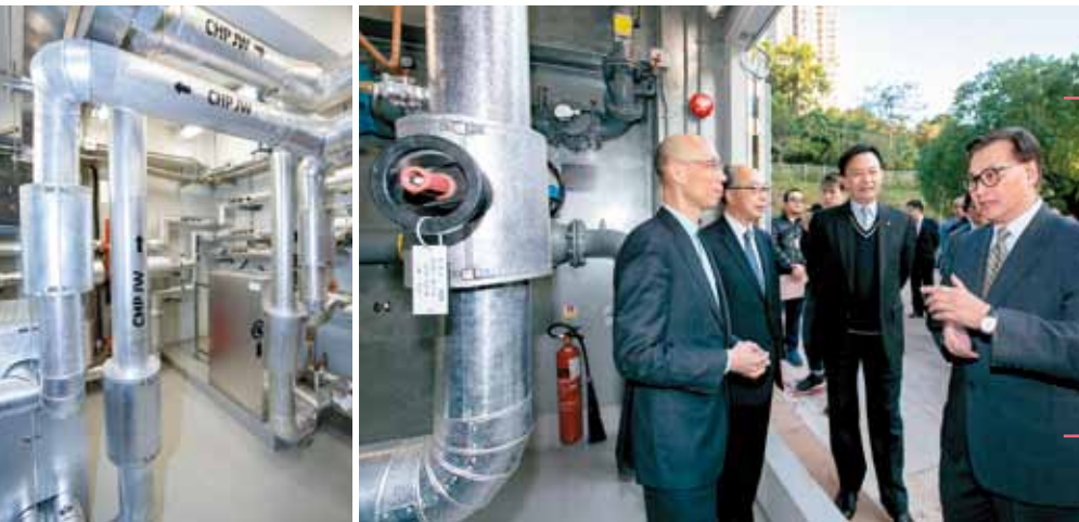
Towngas Managing Director Alfred Chan (right) explains the combined heat and power (CHP) system to Secretary for the Environment Wong Kam Sing (left) at the launching ceremony of the CHP system at Alice Ho Miu Ling Nethersole Hospital.
