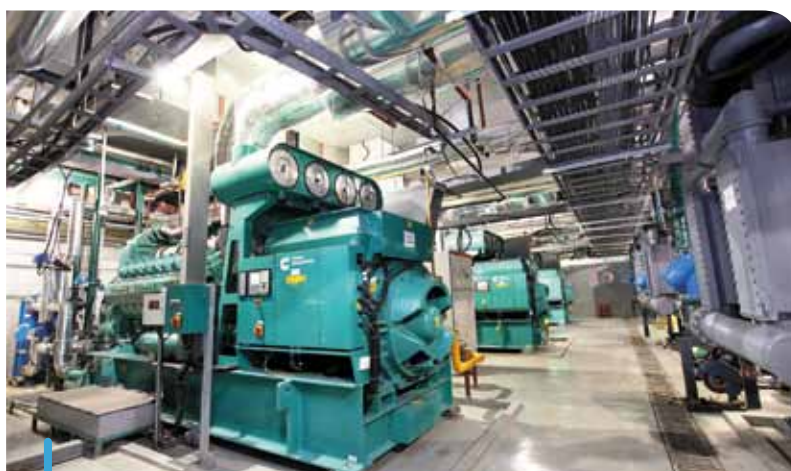
A combined cooling, heat and power system fuelled by natural gas is installed at a data centre in Nanjing, Jiangsu province to enhance energy efficiency.
